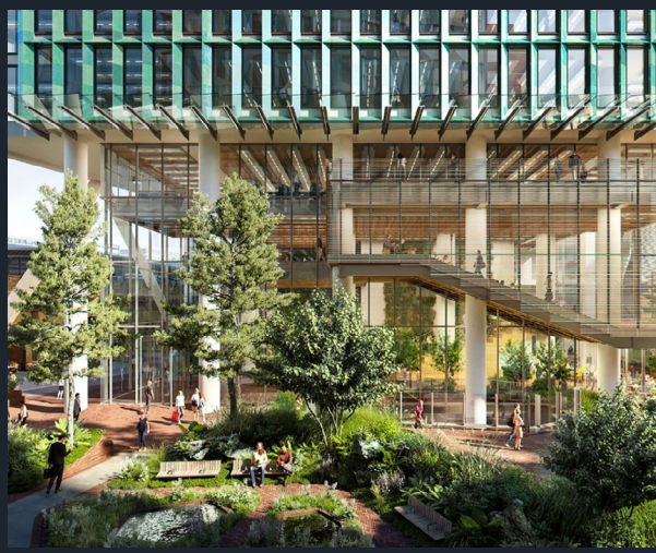
EDGE, London Bridge, London ©EDGE
