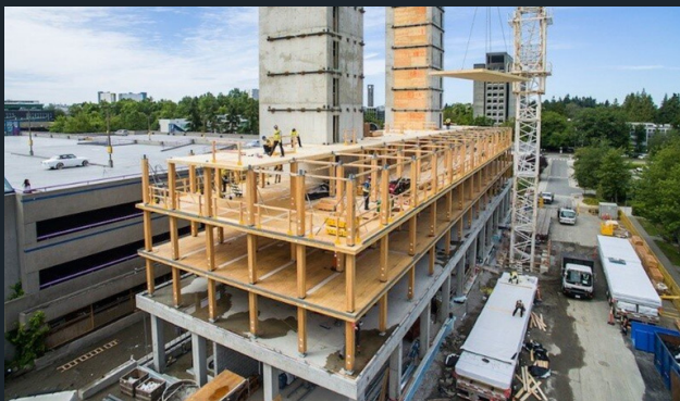
Brock Commons, British Columbia @csengineermag.com
