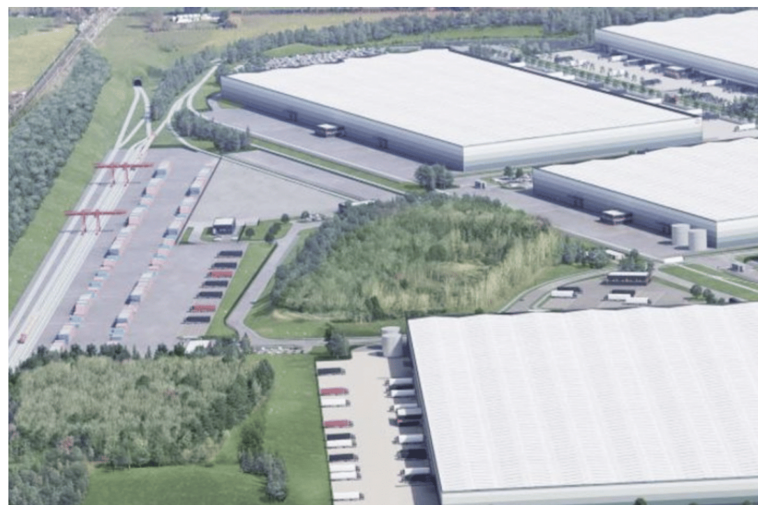
SEGRO and Maritime Transport agreed terms to double the rail freight capacity at SEGRO Logistics Park East Midlands Gateway in June.
